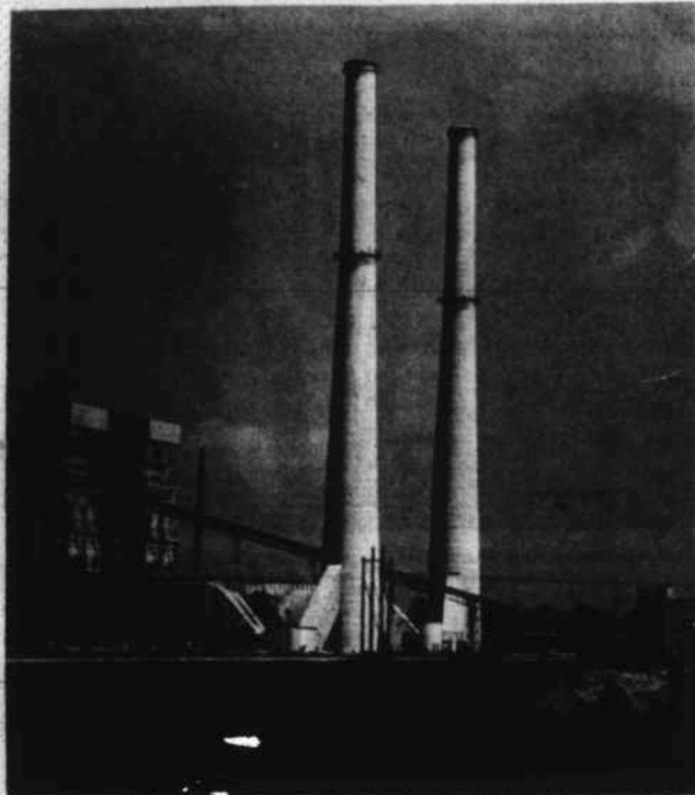
The twin units of the Fayette Power Project near La Grange could produce at least 60 percent of the Lower Colorado River Authority's energy needs this summer. Newly built Unit 2 was put into commercial operation May 21. FPP is co-owned by and produces equal shares of electricity for LCRA and the City of Austin. Photo by Joe Irvin.
